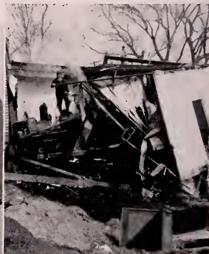
BULLDOZER MOVES IN
